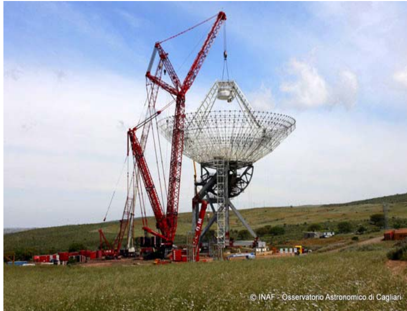
Figure wp14.1: lift of the entire primary mirror support structure
